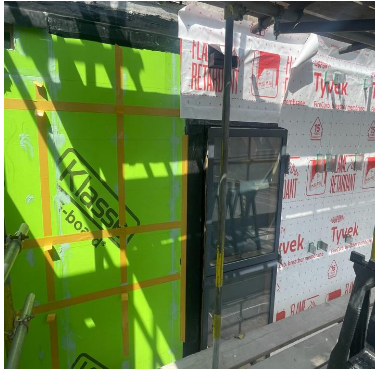
EPDM b2nd layer boarding and Tyvek ongoing
