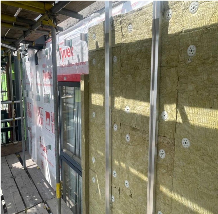
Insulation and helping hands on going
