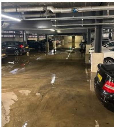
The garage beneath Hebble Wharf can be the first place where a water leak is detected, either from the floors above, or from pipework running along the roof of the garage. Occasionally, when ground water levels are exceptionally high the ground water can also find its way up through joints in the floor resulting in some standing water in the garage.
