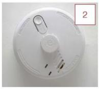
Smoke detectors (Picture 1) are installed in various locations including bedrooms and hallways, with a Heat Detector (Picture 2) in the kitchen. Both types are mains operated with a back-up battery. Each unit should be tested regularly by pressing the TEST button and batteries replaced when necessary. If the detector beeps once every 60 seconds, the battery needs replacing.
